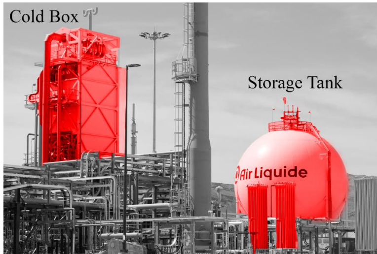
Figure 19.21: Visual aid to demonstrate proximity of cold box and storage tank currently in use at Air Liquide.
